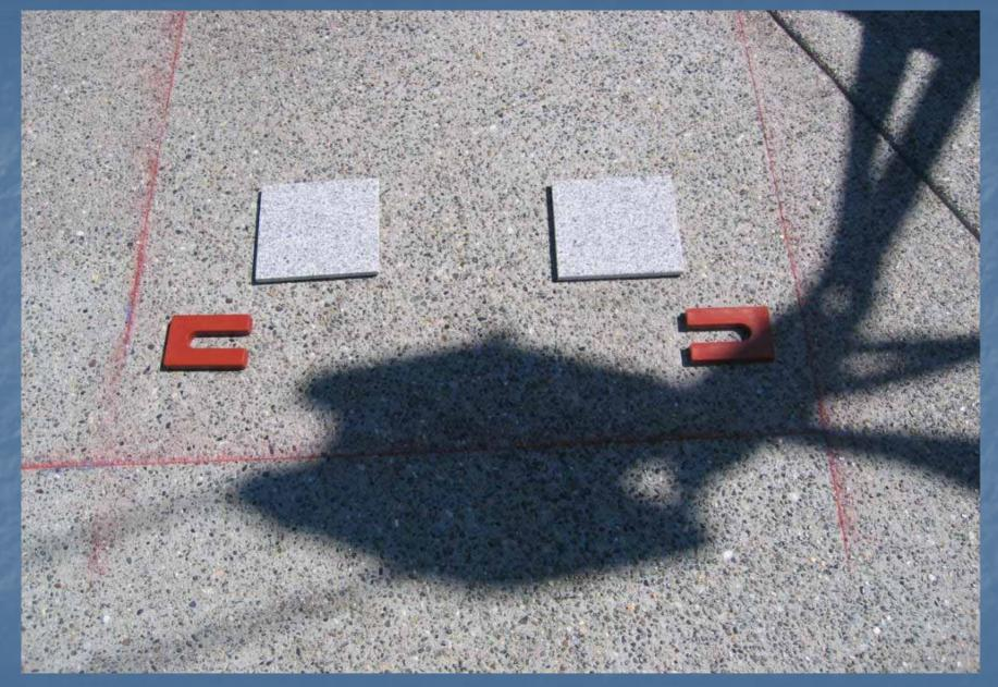
Position of shims and tiles so that crane straps can be removed.
