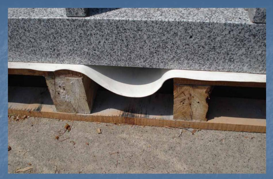
Remove the protective rubber under the columbarium for the lifting straps.
