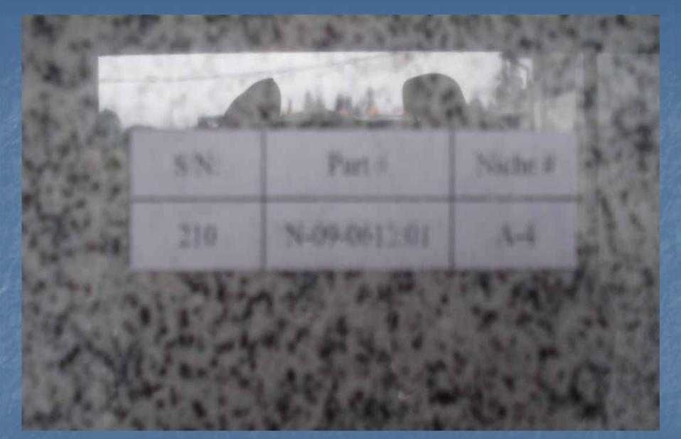
• Each niche has a label on the back wall with a serial number and niche number. Each niche panel has a corresponding number.
