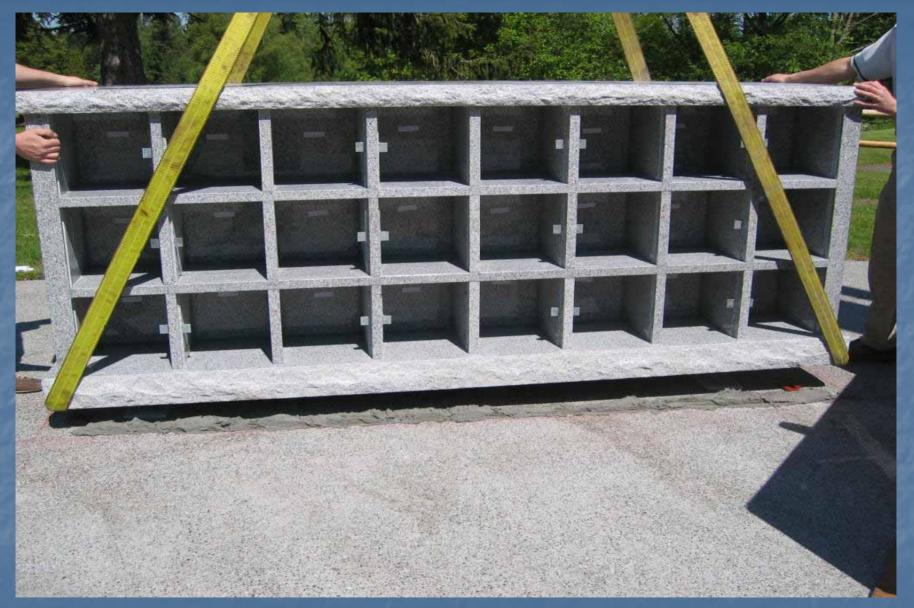
Set columbarium into position. Notice straps are on the outside of the shims for easy removal. Line up with plumb lines.
