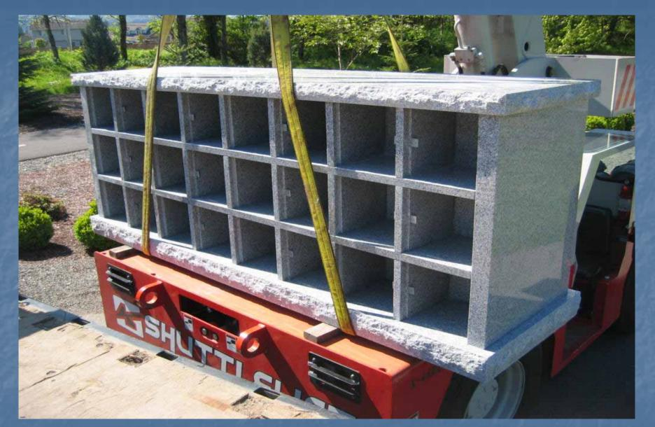
Set the columbarium on the front of the crane to transport into position. Note the wood set down to eliminate the bottom from sitting directly on the crane top.
