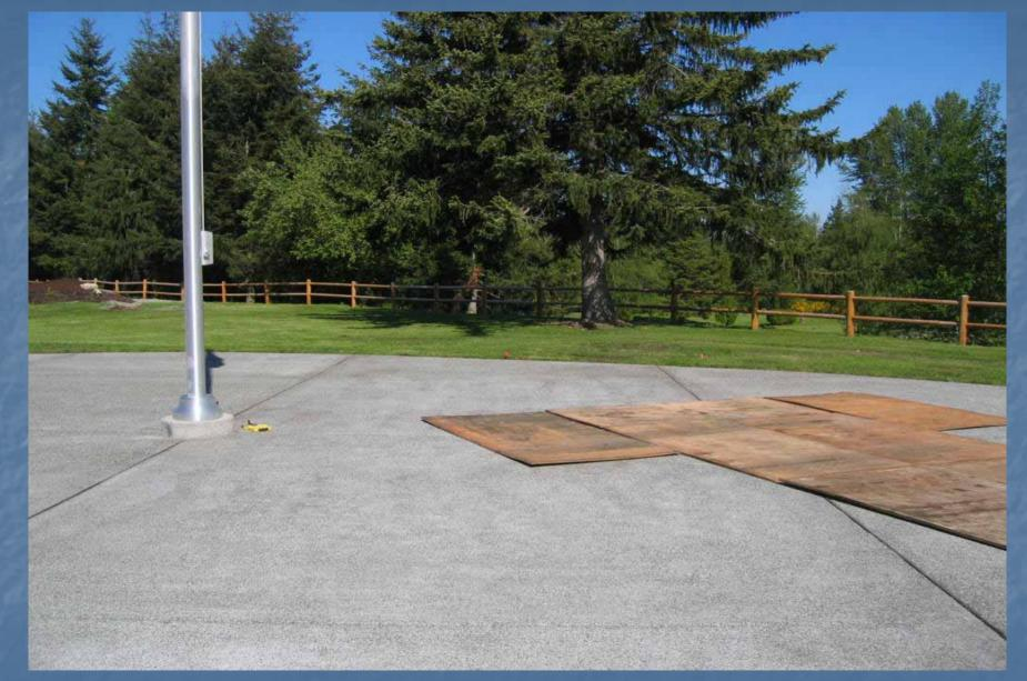
Plywood was set down to prevent tire marks on the new cement while doing the installation.
