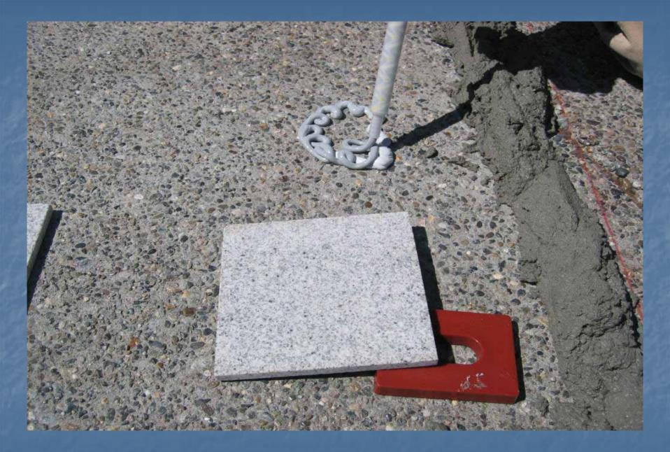
Spread epoxy on cement and the tile.
