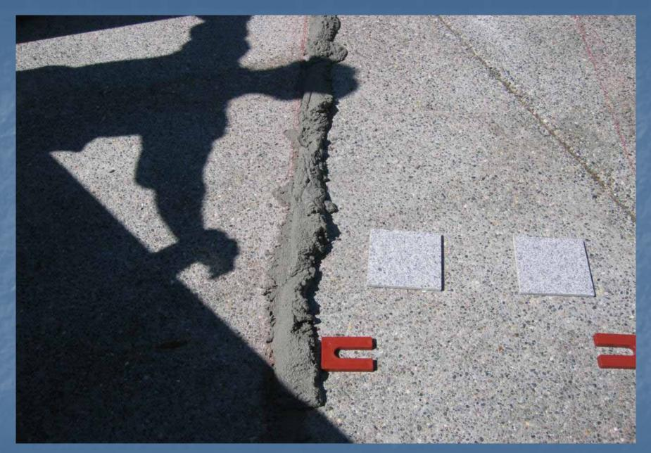
Run mortar mixture along front and back edge.
