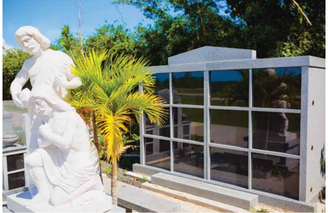
The first of several possible community mausoleums (unless a family decides to buy all 12 crypts) on the Saints Corridor at Guam Windward Memorial. Many of the alcoves just have foundations poured and are available for development as the family desires.
